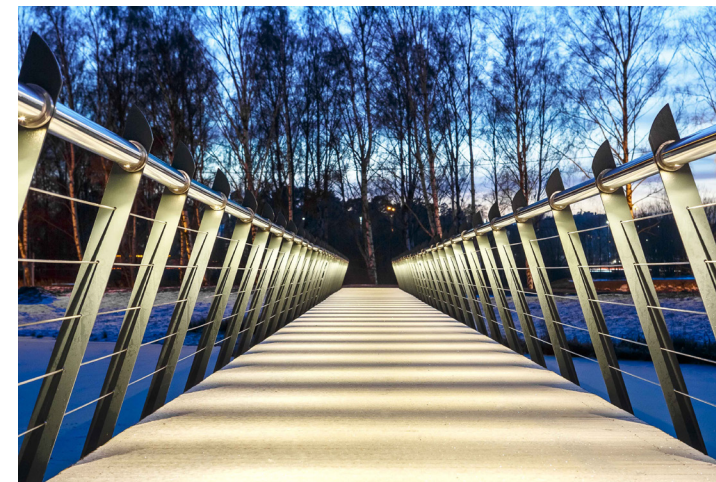
Example Image of Pedestrian Bridge
