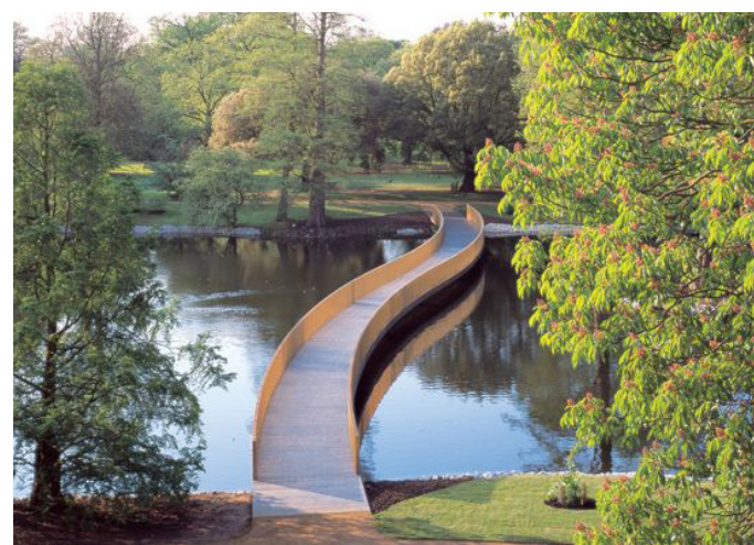
Example image of Pedestrian Bridge
