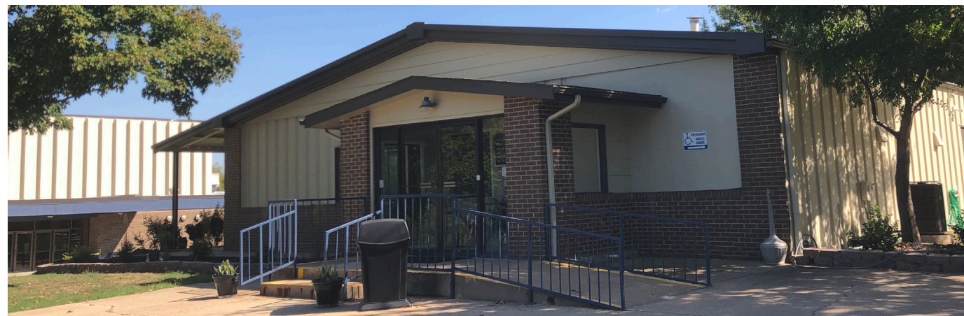
Existing view of ICC Administration Entry (North)
