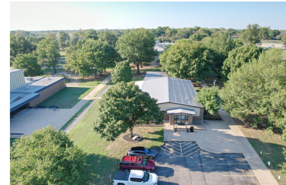
Aerial image of ICC Admin. Building
