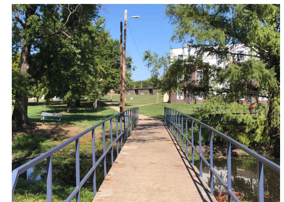
Existing image of ICC Pedestrian Bridge
