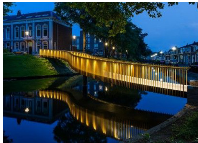
Example Image of Pedestrian Bridge
